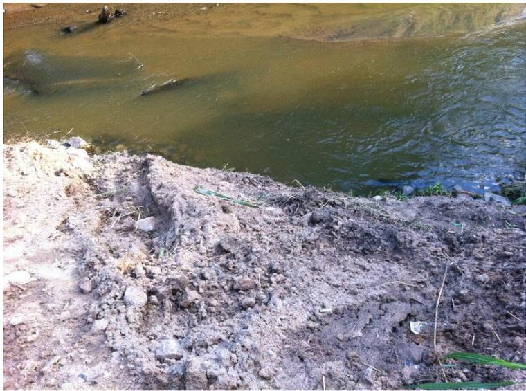
DeKalb County construction site on South River without silt fencing
